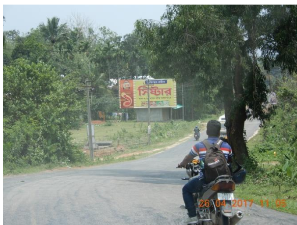
Hoardings located within 10 m from edge of the carriageways which is not conforming to IRC 46 (1972) "Policy on Road Side Advertisements" between Km 8/200 to Km 10/000.
