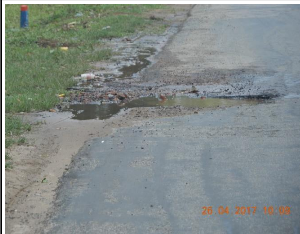
Poor Drainage Mechanism having led to Pavement Distress development during rainy season leaving the road water logged between Km 0/000 to Km 1/200.
