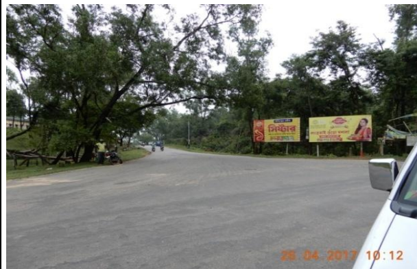
Major junction with Poor Road geometrics requiring redesign conforming to IRC.SP-41 (1994) coupled with absence of Traffic Calming Measures Minor Road Junction and Absence of Over Head Gantry / Shoulder Mounted Sign on Major Road @ Km 1/200.
