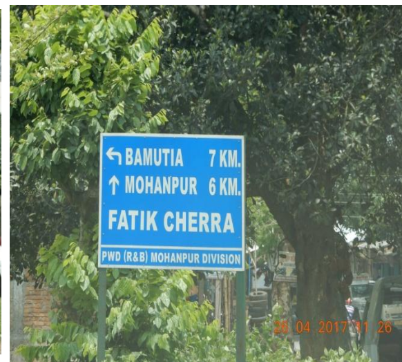
Non-standard Direction Information Sign between Km 10/000 to Km 13/600
