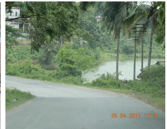
Accident Block Spot at Km 7/100 , (near Lembucherra) Horizontal and vertical curve on water body with sight Distance obstructions due to trees
