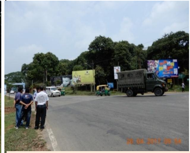
Absence of Segregation Treatment for the Through Traffic bound to Agartala from Durjainagar at Km 0/000
