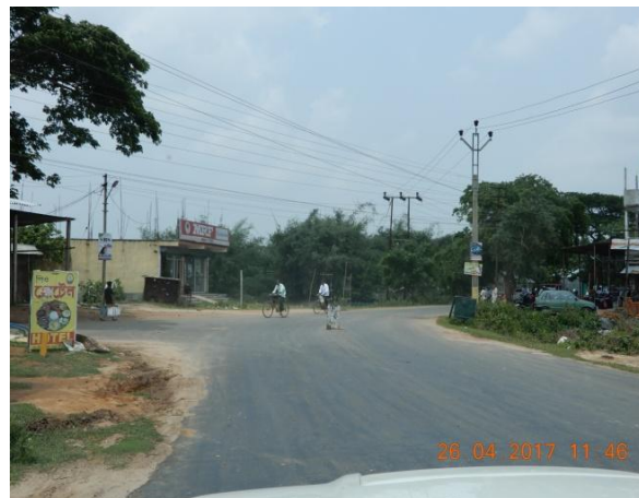
Major junction with Poor Road geometrics requiring redesign conforming to IRC.SP-41 (1994) coupled with absence of Traffic Calming Measures on Minor Road Junction @ Km 17/700
