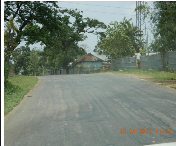
Accident Black Spot at near Km 16/000, series of Horizontal curve with sight Distance obstructions due to trees
