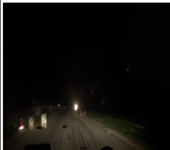
No reflective taps on drums for reducing the speed
