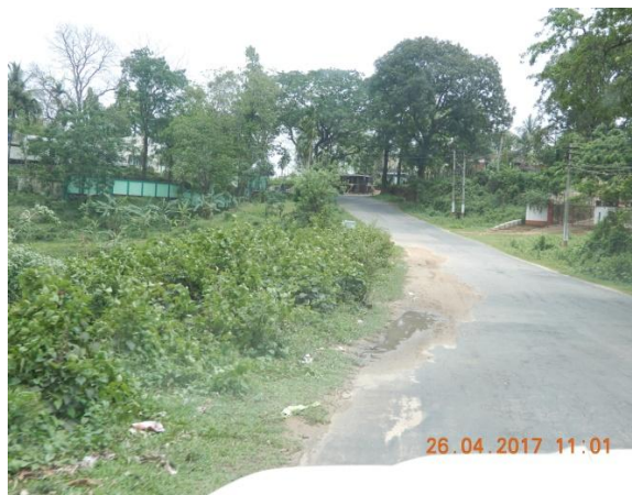
Accident Block Spot at Km 7/100 , (near Lembucherra) Horizontal and vertical curve on water body curve with sight Distance obstructions due to trees
