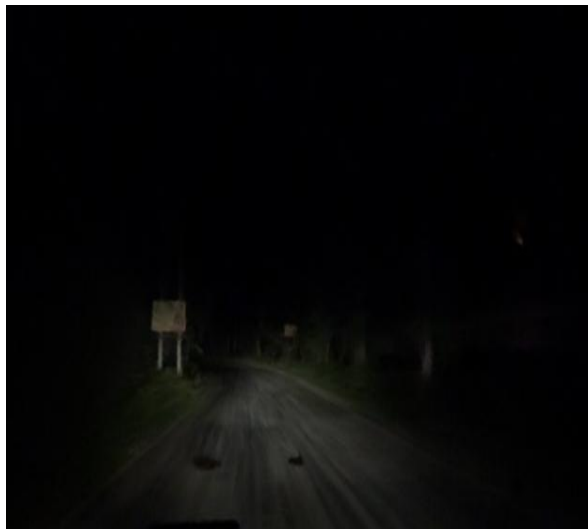
No delineations and chevron signs on curves
