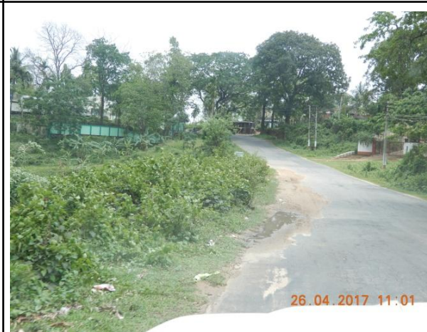
Pavement cracks observed on pavement and heavy sand deposited on pavement it may lead skidding of vehicles between Km 7/100 to Km 8/200
