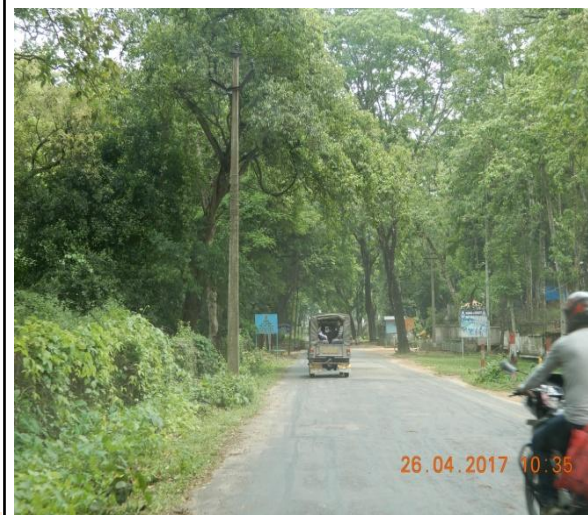
Electric pole and trees without Retro reflective Taps between Km 1/700 to Km 2/500.
