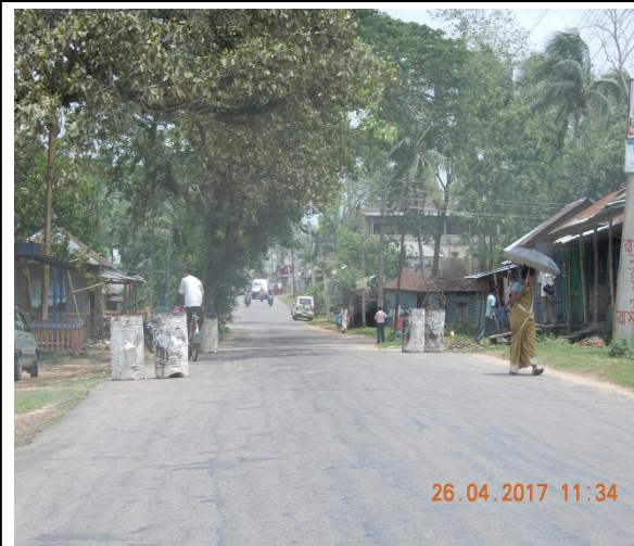
Non-standard Speed Breaker; not conforming to IRC. 67 (2012) between Km 13/600 to Km 17/700
