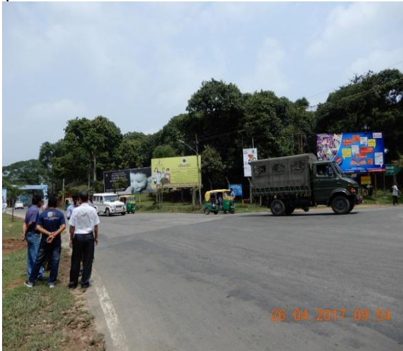
Poor condition of shoulders with on either side with fully grown grass making it unusable by any form of traffic / Pedestrians
