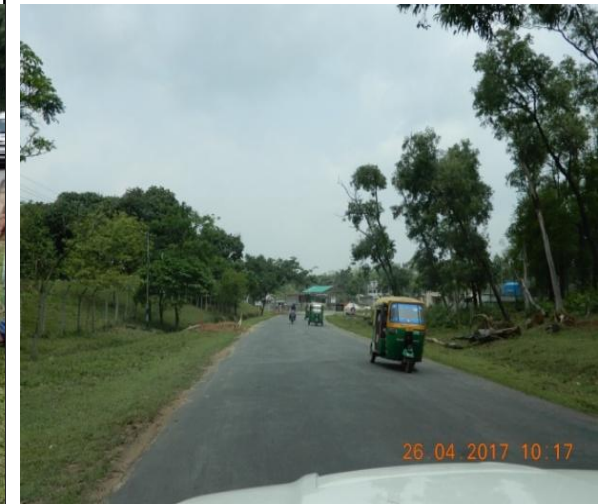
Poor condition of shoulders with on either side with fully grown grass making it unusable by any form of traffic / Pedestrians
