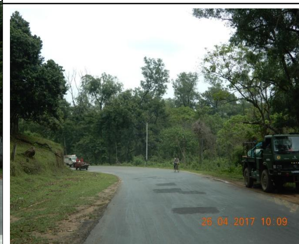
Absence of 'Curve Ahead' Warning Signs and 'Chevron Signs' and trees obstructing the Sight Distance at the horizontal curves between Km. 0/000 to Km. 1/200 on LHS & RHS
