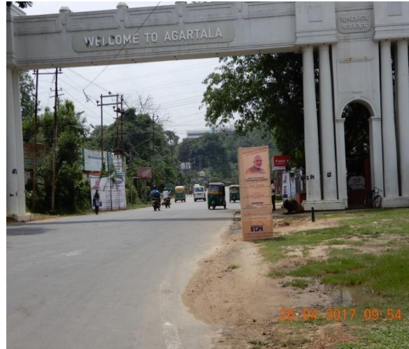
Absence of Segregation Treatment for the Through Traffic bound to Agartala from Durjainagar at Km 0/000
