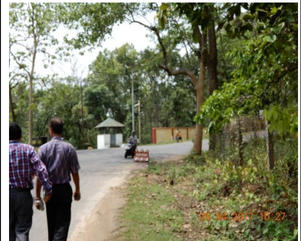
Accident Black Spot at Km 1/700, Horizontal curve with sight Distance obstructions due to trees
