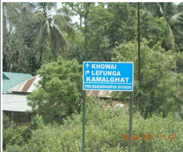
Non-standard direction Sign board; not conforming to IRC.67 (2012) between Km 10/000 to Km 13/600.
