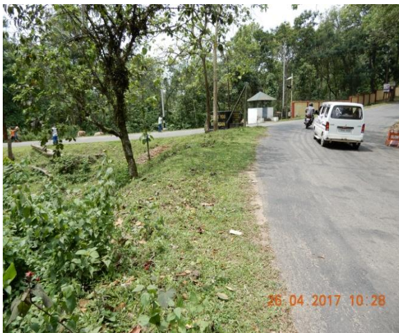
Accident Black Spot at Km 1/700, Horizontal curve with embankment without crash barrier
