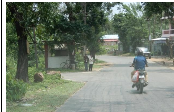
Absence of Side Road Left' Warning Sign coupled with Direction Destination Sign for the Minor Road Crossing coupled with Absence of Speed Calming measures on the minor road merging with Project Corridor - Many such between Km 10/000 to Km 13/600.
