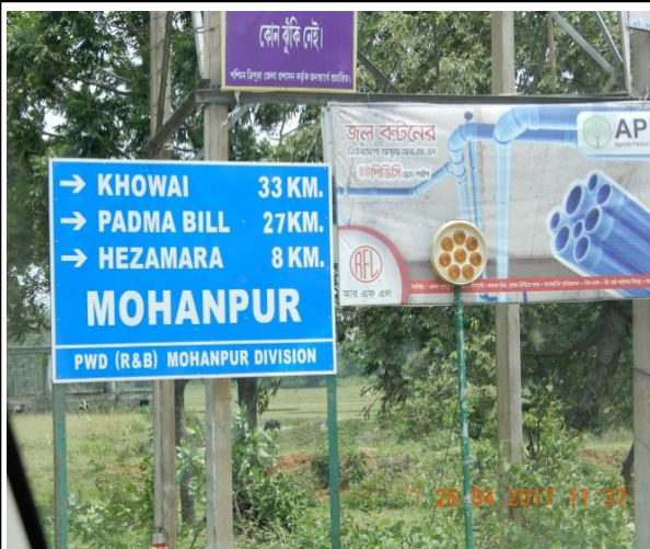
Non-standard Direction Information Sign board; not conforming to IRC.67 (2012) between Km 17/700 to Km 20/000
