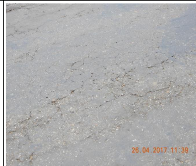
Pavement cracks observed on pavement between Km 17/700 to Km 20/000
